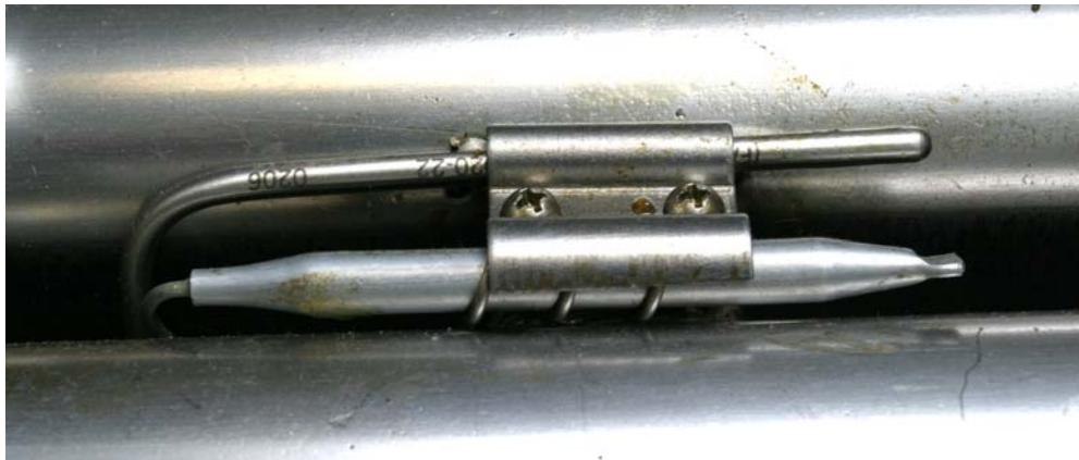
Typical high-limit/sensor probe locations and mounting hardware.
