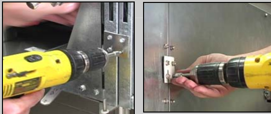
Figures 7,8: Use screws to attach securing brackets. Ensure the rear bracket screws go through the vertical stiffening channel
